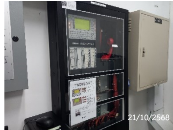
Fire Alarm Control Panel
