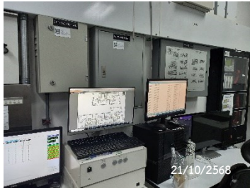
Graphic Annunciator Fire Alarm System
